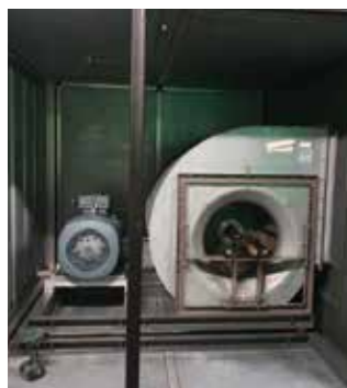
One of the large recirculation fans before and after renewal. Photos: Lufttechnik AG Wädenswil.
