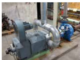
Left: the old pump with the original direct current motor, cooling and extraction. Right: the new pump in a housing. Photo: Topmotors
