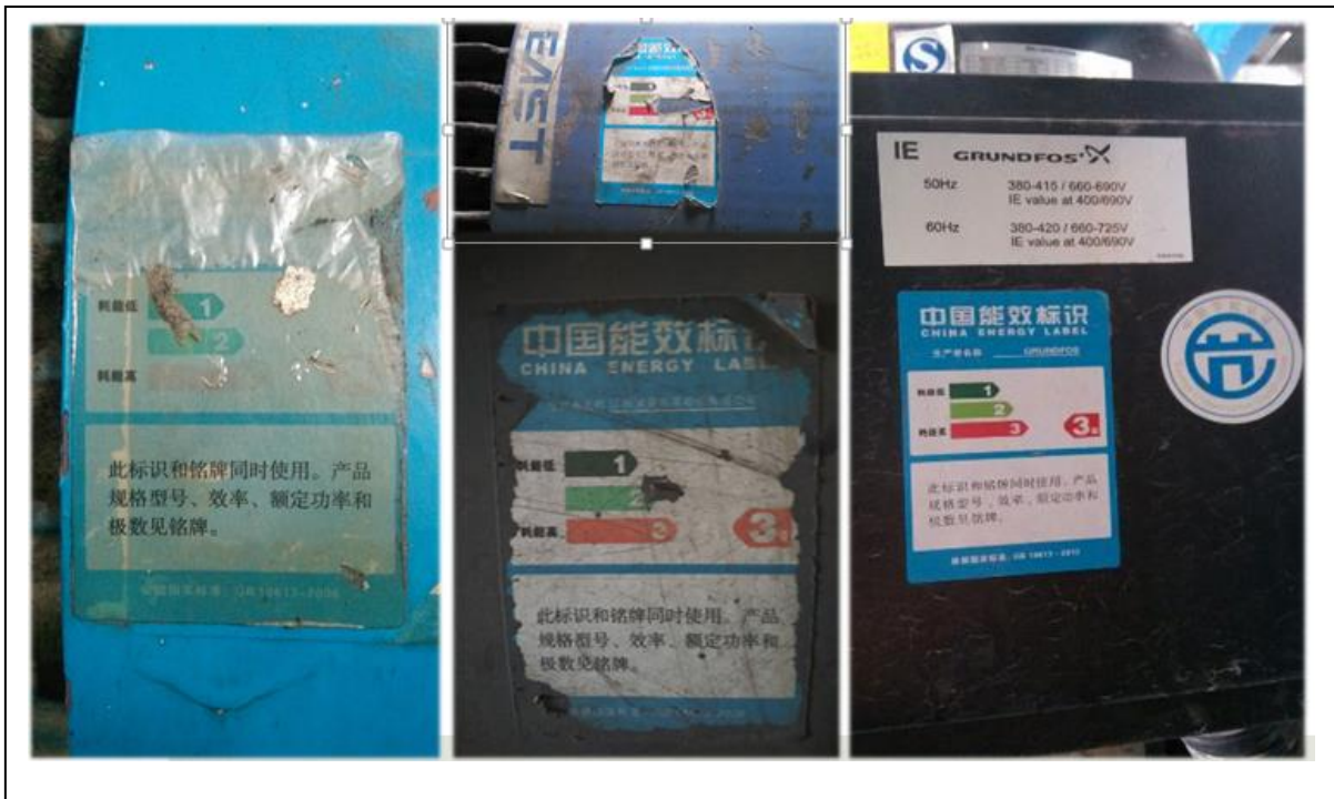
Figure 5 CEL of motors in factories, Jiangsu province, China
